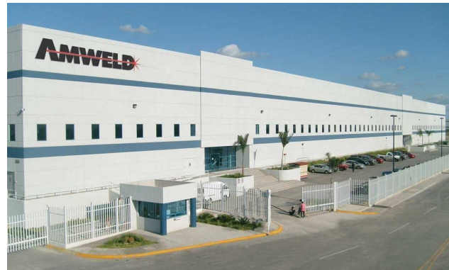
Amweld's 200,000 square foot facility operates with state-of-the-art equipment, technology, and a cost-effective mind-set.
